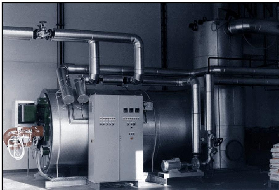
**Figure 4.27: Unit for direct-flame incineration with afterburner**
